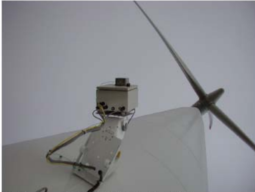
Figure 1.2. Thermal camera mounted with a pan/tilt head on the A2 offshore turbine at Nysted wind farm.
